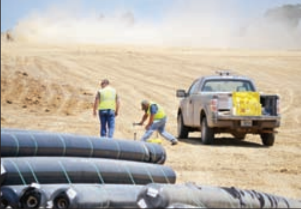
Neal Robertson, highway engineer, and Joe Quermous, engineer assistant, stake out a portion of the highway behind some material that is used as a base for the roadway and its right-of-way.
