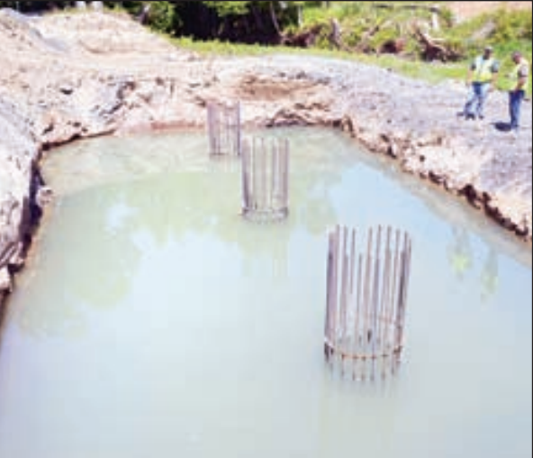
Highway workers examine the location of pillars that will support the new highway's bridge across Livingston Creek near Fredonia.
